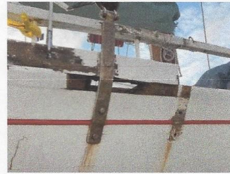
Even well maintained wooden boats need repairs This example replaces 10 feet of log rail and decking
