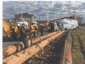
Local old growth loblolly pine logs are being prepared to replace Nathan's 27 year old mast and boom.
